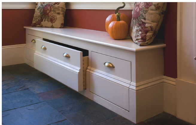
The baseboard trim profile continues across the built-in bench in the mudroom for a traditional look.
